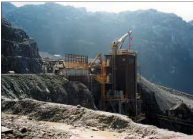
Fig. 2: Semi-mobile crushing plant Abb. 2: Semi-mobile Brechanlage
