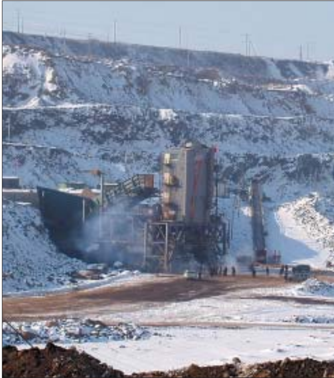
Fig. 16: Completing the relocation job
